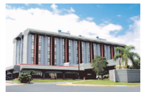
HOSPITAL PAVIA, CAGUAS 787-653-3434
